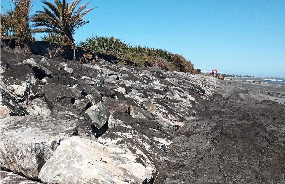
Completed emergency rock works
