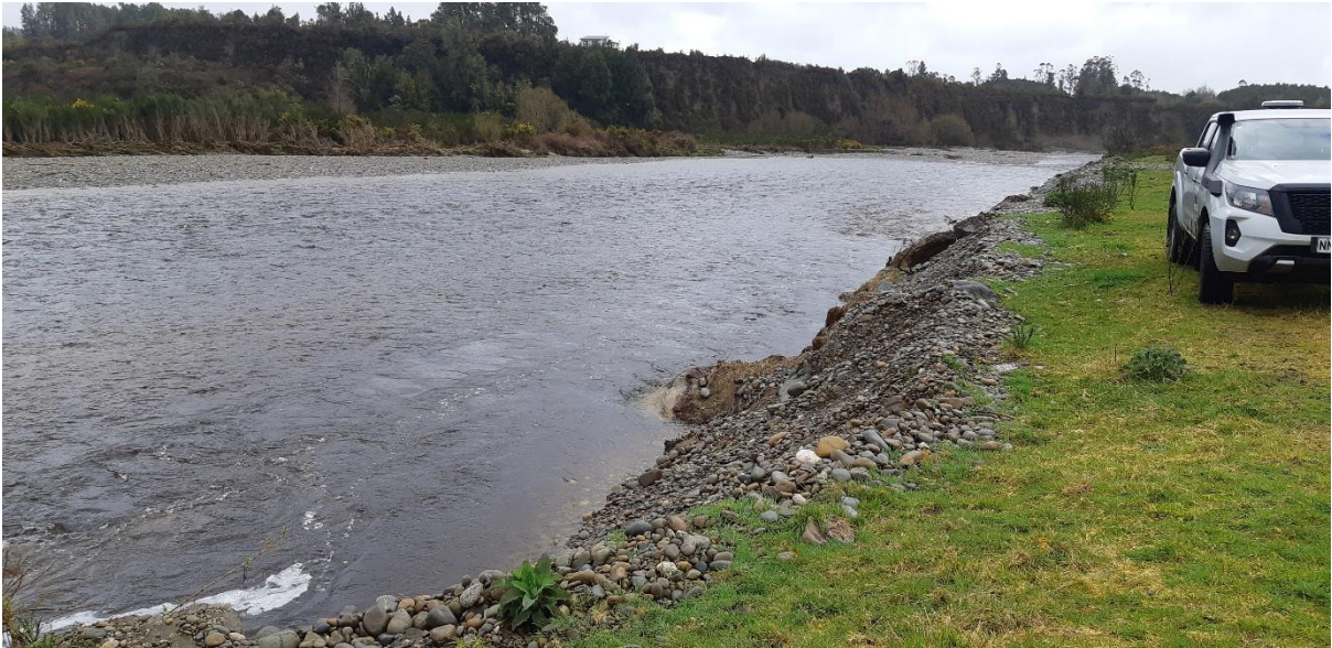
Photo 2: Looking downstream where the gravel bund has been removed.
