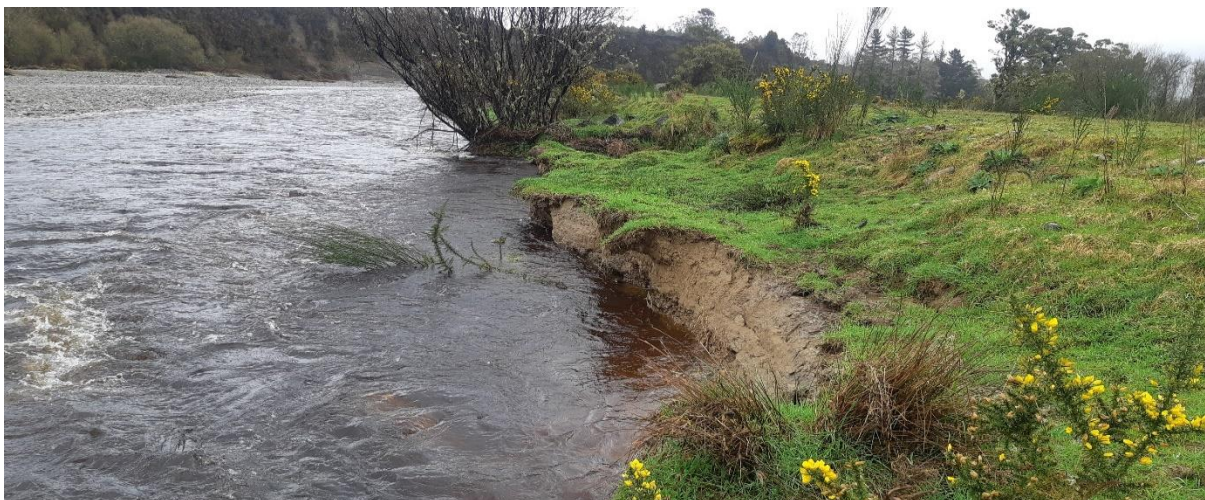
Photo 1: Looking downstream at erosion of one of the unprotected berms
