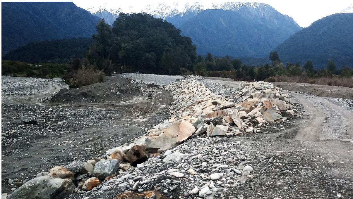
Looking up stream from Milton & Others Stopbank
